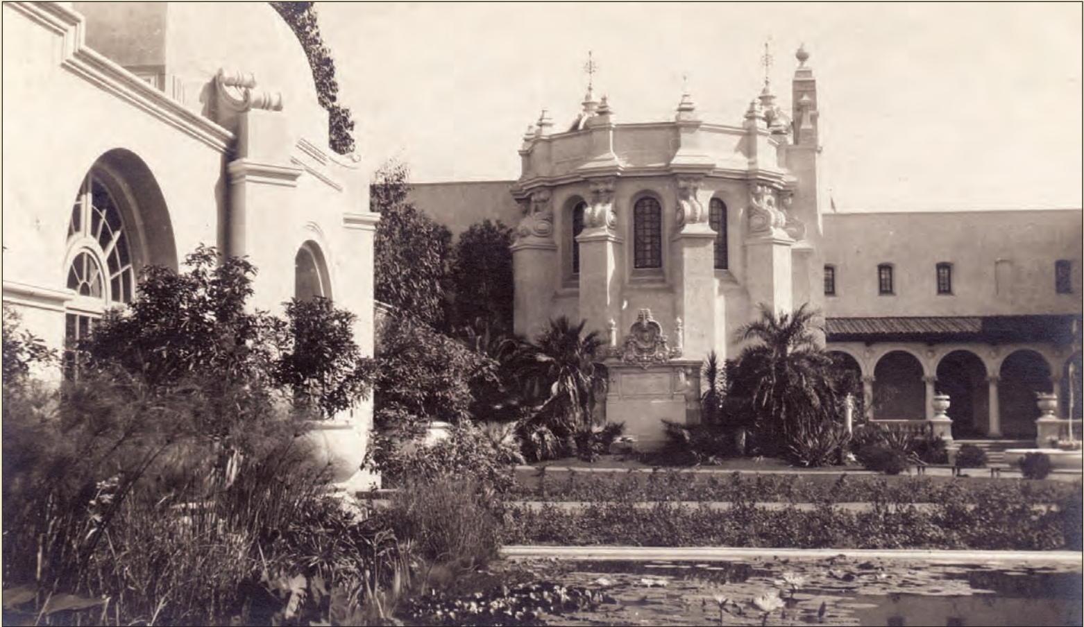
West apse of the Food & Beverage Building and Serra Memorial were omitted from the 1971 reconstruction.
